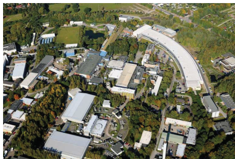
Figure 1: Aerial view of the new experimental hall of PETRA III which was built from 2007 to 2008.
