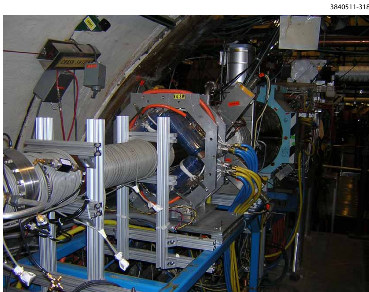
Figure 2.131: View of solenoidal field windings on the L3 straight section vacuum chambers.
