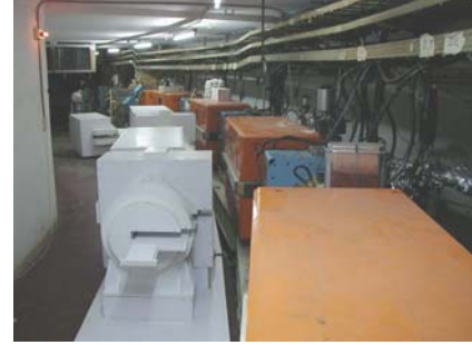
Figure 10: The wood “magnets” in the BEPC tunnel
