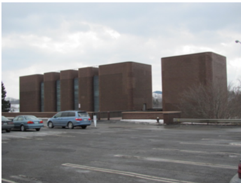
Figure 4.4.6: The Wilson Lab cooling towers.
