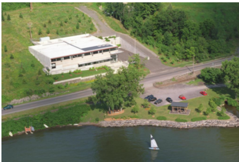
Figure 4.4.5: The Cornell Lake Source Cooling (LSC) plant.
