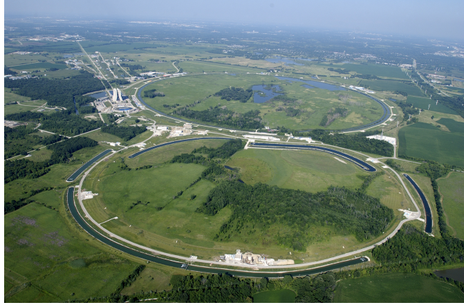
Figure 3.1: Areal view of the Fermi National Accelerator Laboratory.
