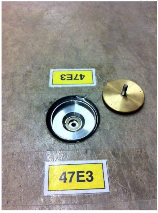
Figure 2.120: Floor target with cover removed.
