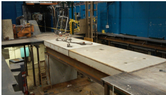
September 16: New bridge over CLEO pit
